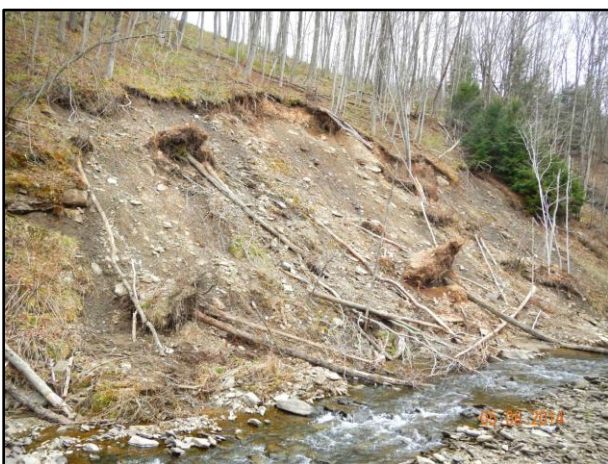
Portion of bank failure in early 2014, looking upstream.
